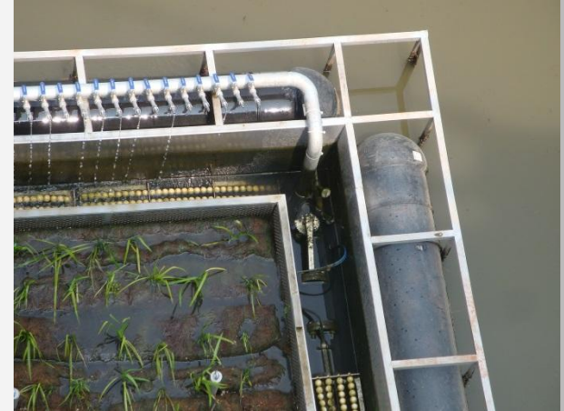
Clogging of water input
