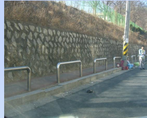
Inappropriate crash barrier
