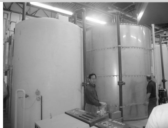
1 st Anoxic tank + Aerobic tank
