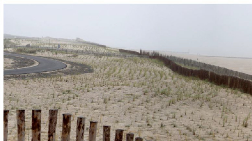
Sand-packed dyke near Nieuwvier, which has created a new recreational beach and dune landscape. (Photograph: Melle Wierman/ANX).
